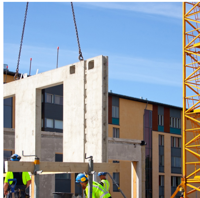
3. Indicate the sequence of erection of pre-cast panels to allow for safe demolition.
